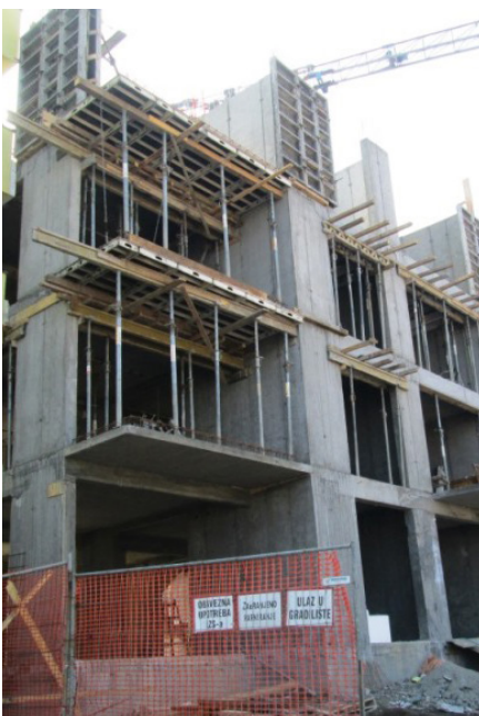
Zgrada u Tuzli, mart 2017 / Building in Tuzla, March 2017
